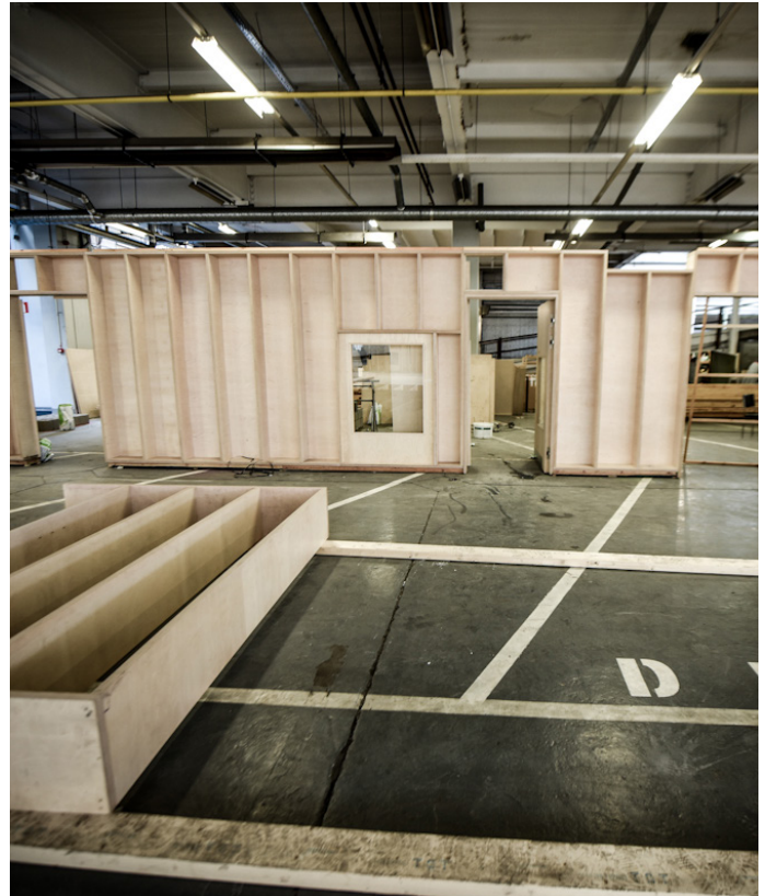
Installation of panels at Kanal Foundation
