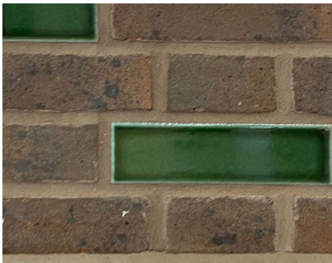
Flemish bond with glazed brick flair mock-up
